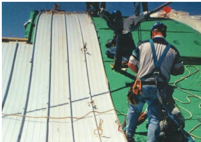
RoofShield installation at Detroit Metropolitan International Airport
