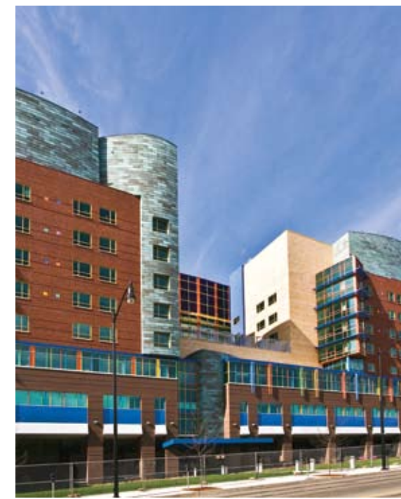
Children’s Hospital of Pittsburgh, UPMC, Pittsburgh, PA photo: Alexander Patho Photography
